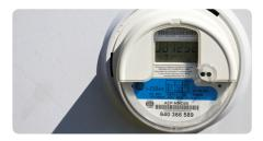
A utility meter measures both energy used from the electric grid and excess energy produced from your solar panels.
